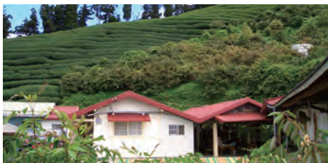
The reconstruction of 100-year three-section compound becomes guest room with historical flavor now
