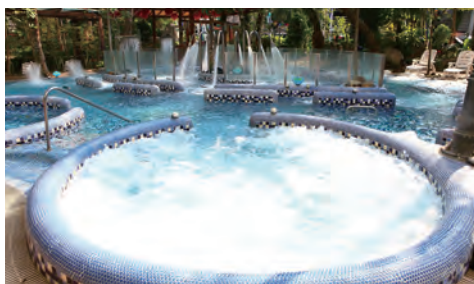
Outdoor spa equipment
